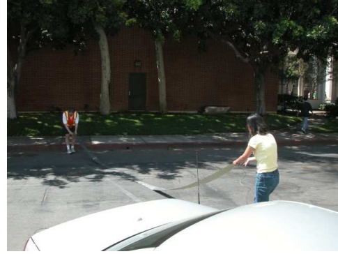
Figure 12: ILD being installed on the roadway
