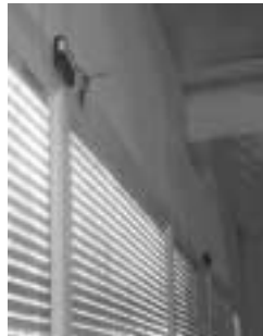
Fig. 7. Beacon deployment in the UCLA Laboratory for Embedded Collaborative Systems (LECS). Motes are attached to the ceiling tiles.
